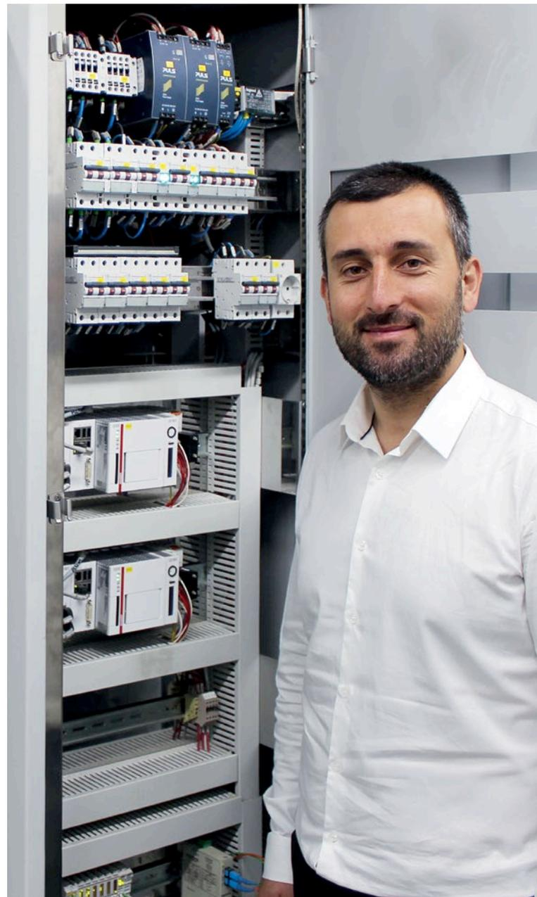
A total of 84 Beckhoff CX2020-0121 Embedded PCs are used in this project as a gateway control system in 42 rail stations.
