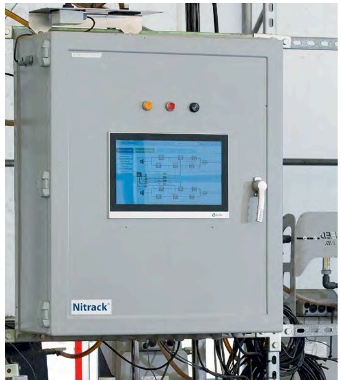
Nitrack® from EOSi integrates the first PC-based controller that is used for monitoring biological nutrient removal in wastewater treatment.
