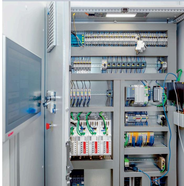
The view inside the control cabinet shows the Beckhoff C6030 ultra-compact Industrial PC and the inline connected EtherCAT Terminals (center right) as well as the AX5000 Servo Drives (center) and the 12-inch CP2912 multi-touch Control Panel (left).
