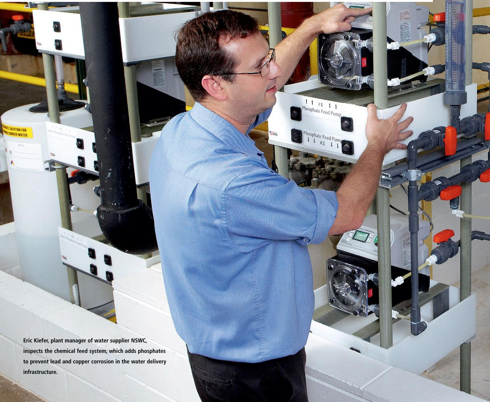
Eric Kiefer, plant manager of water supplier NSWC, inspects the chemical feed system, which adds phosphates to prevent lead and copper corrosion in the water delivery infrastructure.
