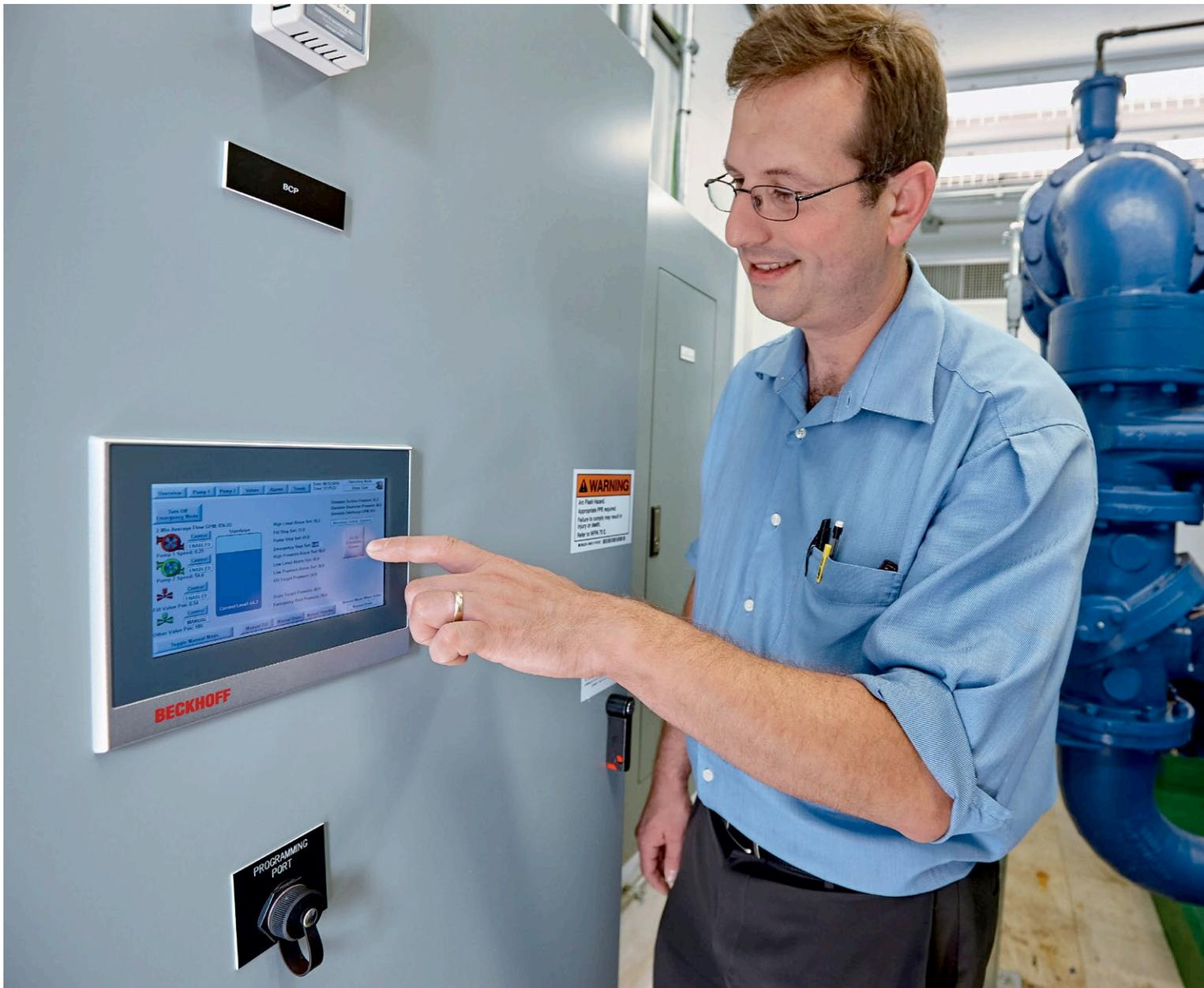
The pumping station is controlled via a CX2020 Embedded PC with directly connected EtherCAT I/Os.
