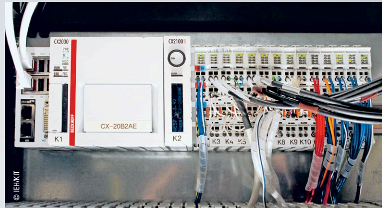
For inverter emulation, the CX2030 Embedded PC enables short control cycle times of 50 \mu s.
