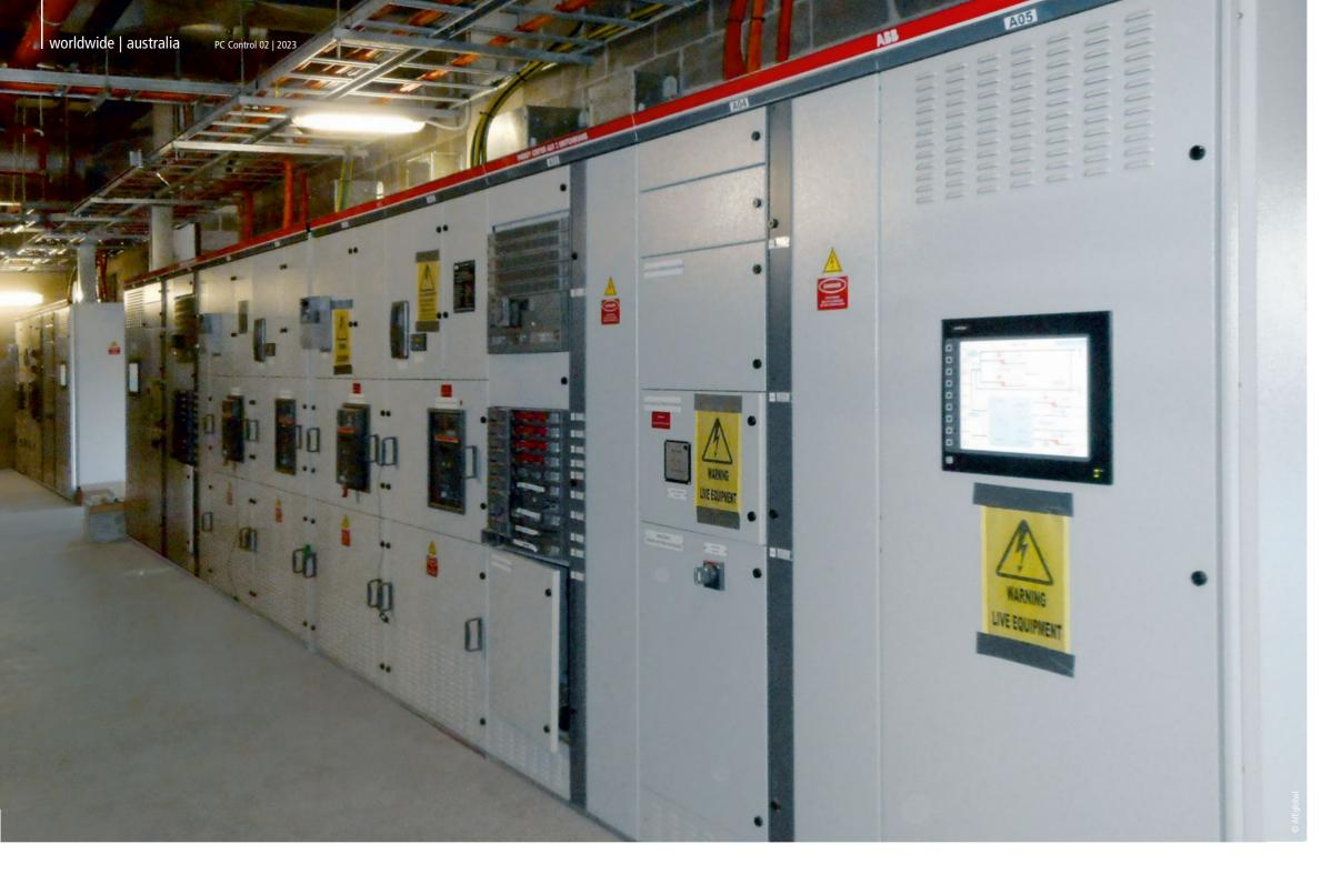
Implementing EtherCAT communications on each generator considerably reduced the wiring requirements and also the central control cabinet size to a single 800 mm tier.
