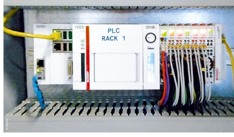
Seven CX2020 Embedded PCs were selected to automate the four 2 MW generator sets, the heat exchangers and the overall plant control system, as well as the connection to the SCADA system.
