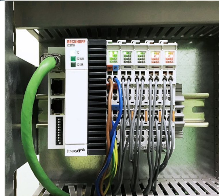
Beckhoff CX8110 Embedded PC with EL3182 analog EtherCAT input terminals for HART-capable field devices
