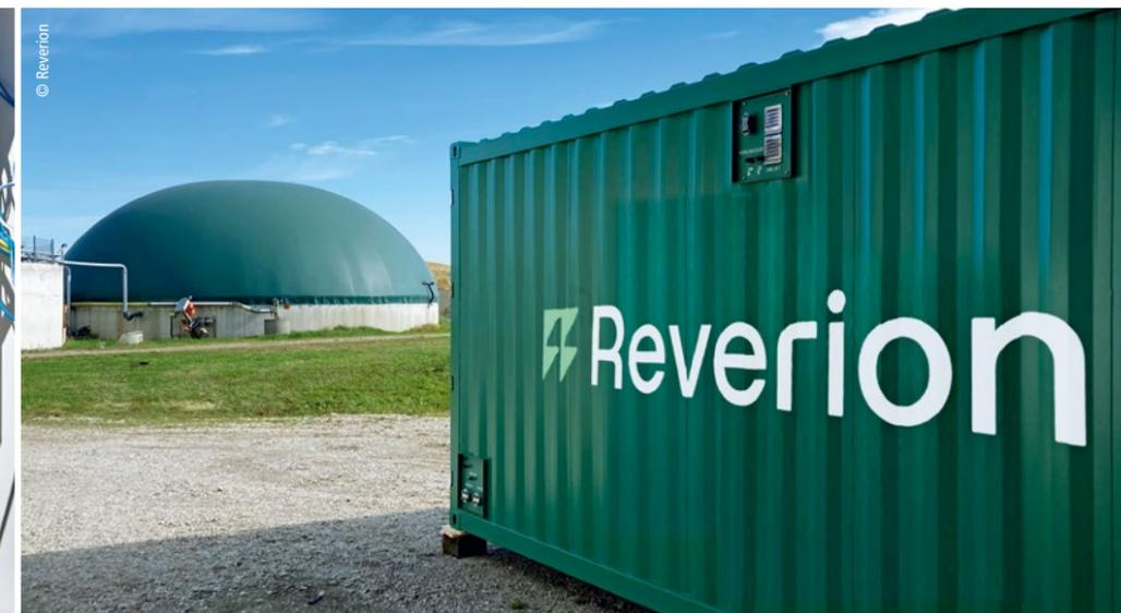
The Reverion biogas power plants are housed in a highly compact container, achieve a high efficiency of 80%, and allow reversible operation.
