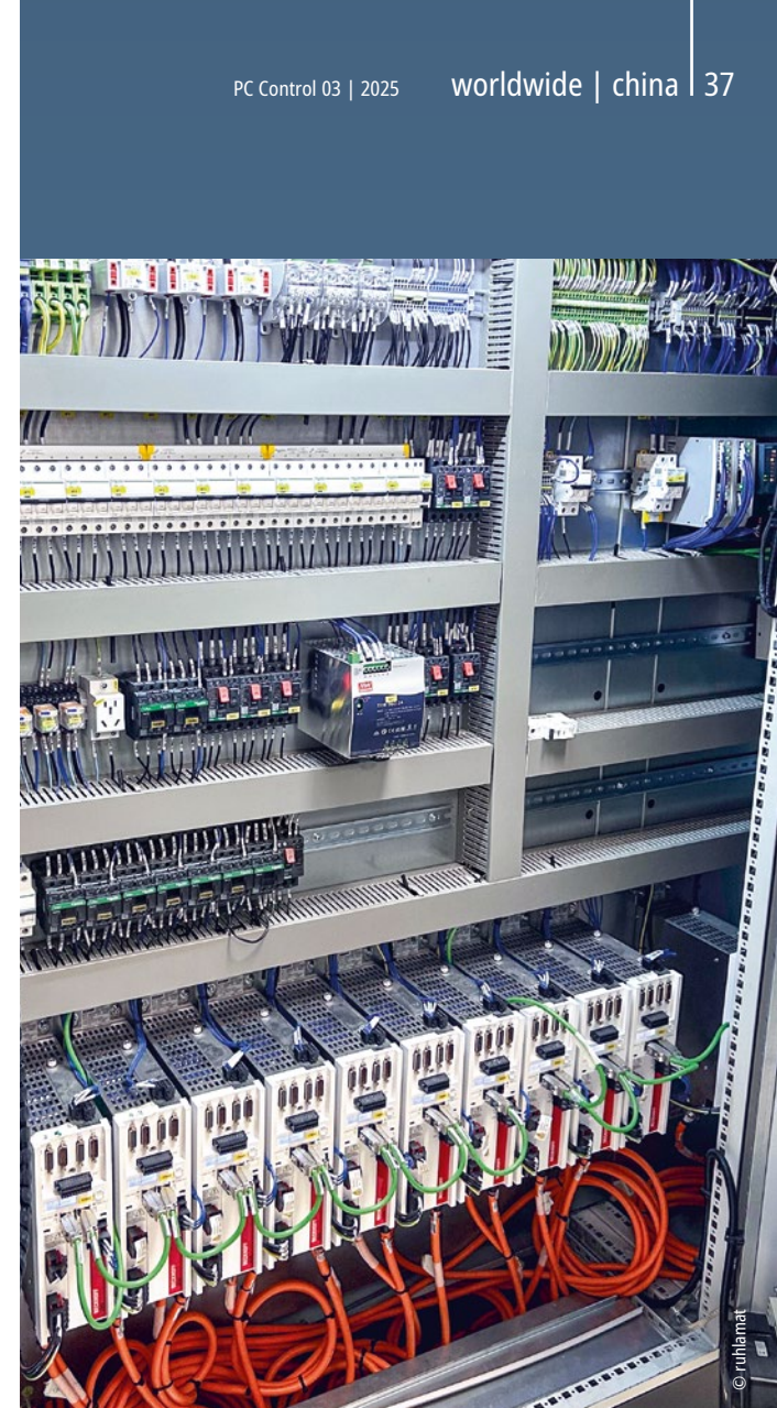
Control cabinet with numerous Beckhoff AX5000 servo drives (below)
