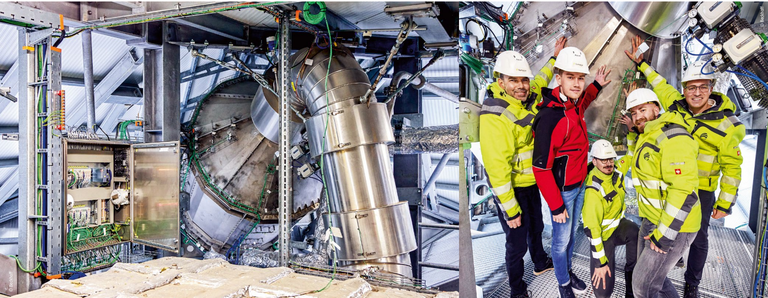
Left: The receiver with 600 kW thermal output and the ceramic energy storage unit (in the foreground) are monitored via numerous thermocouples.
