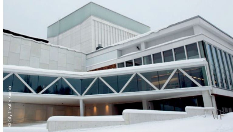
The City Theater in Kuopio, Finland. The building's old and new sections are connected by a kind of bridge that runs from the lobby in the old part along its facade to the auditorium in the new part while forming a protective canopy.
