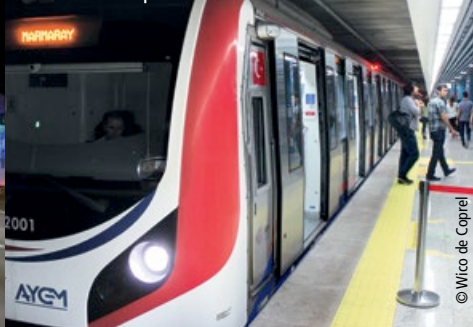
Marmaray rail tunnel, Istanbul, Turkey Wico de Coprel
